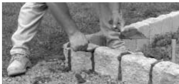
Tooling the joints
