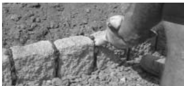
Mortaring joints with mortar bag
