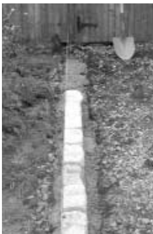
String line for aligning the block
