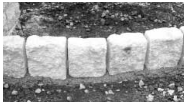
Wet bed application with mortar joint spacing
