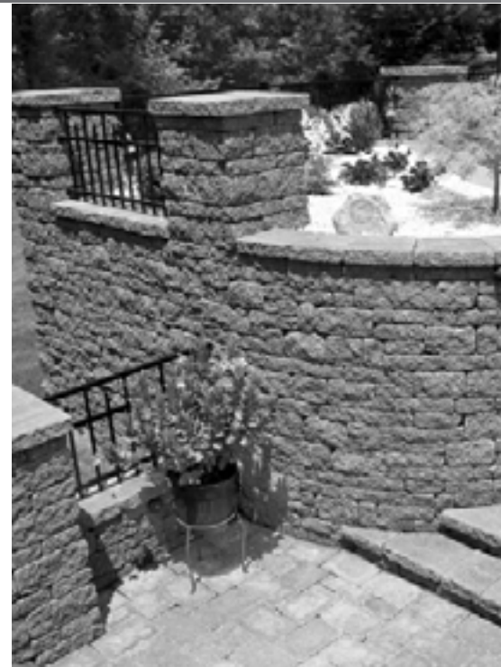
▲ This wall has been engineered due to its height
