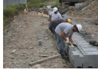
Cleaning debris off units
