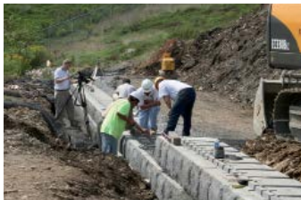
Installing geogrid horizontally
