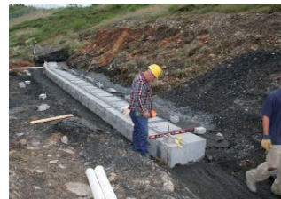
Leveling each unit
