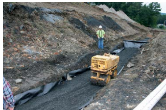
Geotextile and compaction
