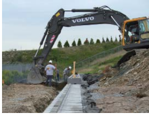
Installing the first course
