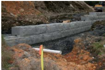
Installing the first course
