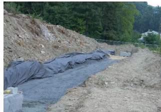
Leveling pad after compaction
